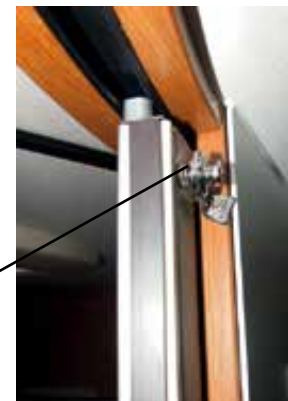
Securing the lamella roller door with spring button lock
