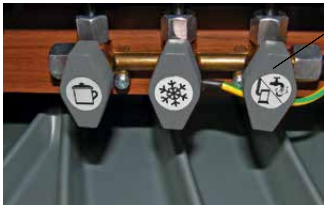
Gas valve, heating = open
