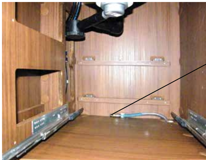
Air-bleed valve behind wash- basin drawer
