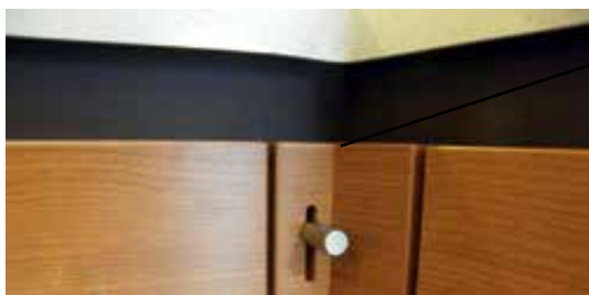
Pin up = telescopic elements unlocked
